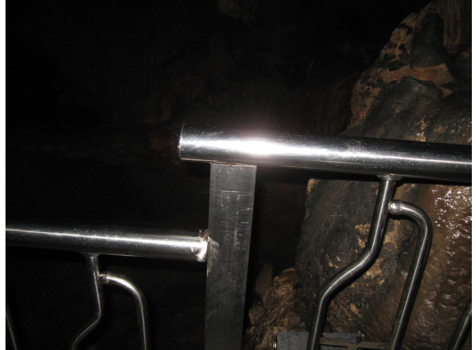
Handrail transition at a step. Neil and I each witnessed several stumbles as a result of the 'vanishing' handrail (above)
