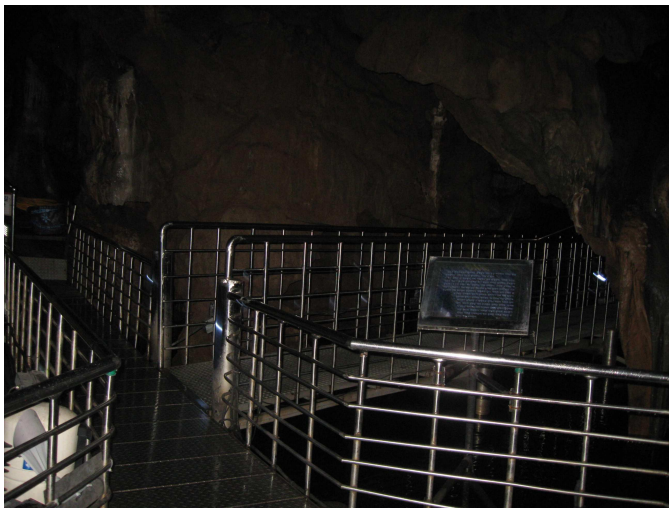
Note the variation in handrail height and the horizontal bars
